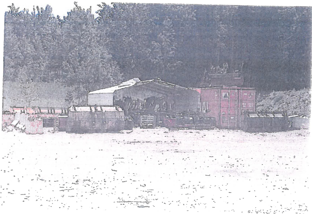
Southwest Corner of Property and Elevation Change
