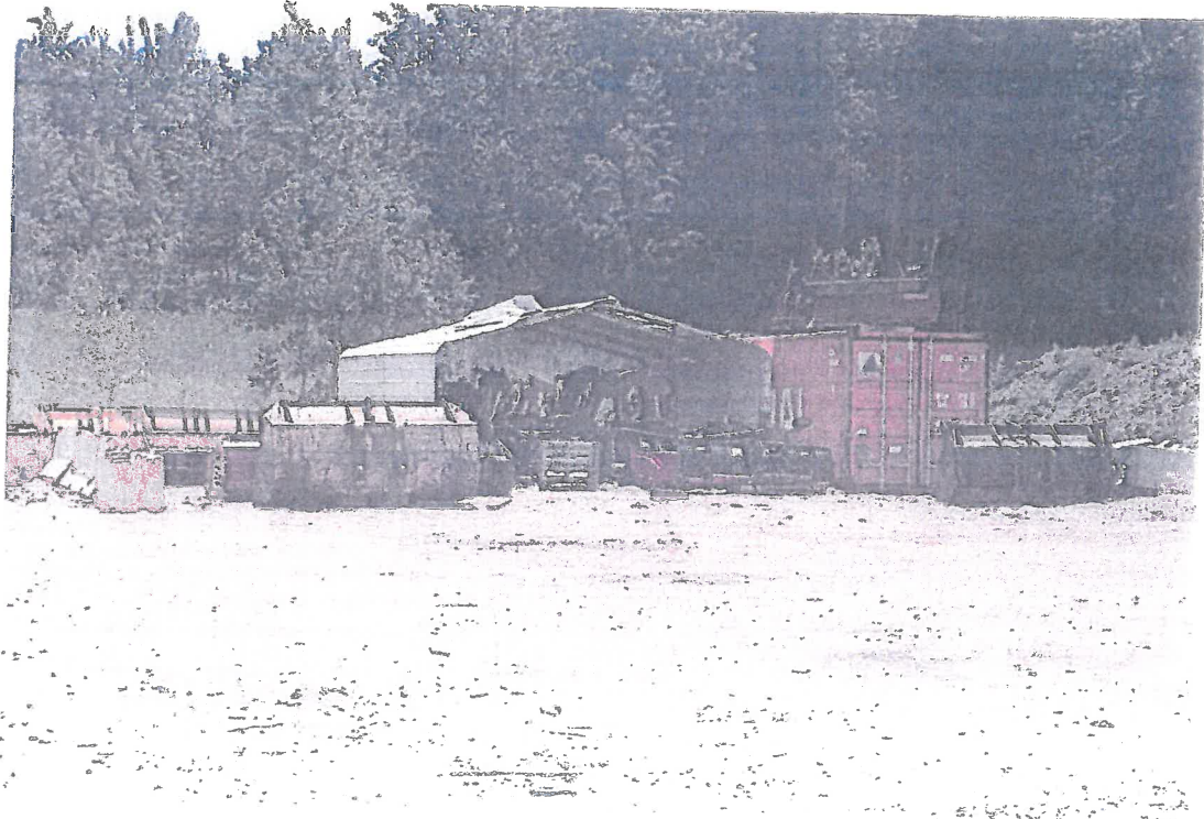
Southwest Corner of Property and Elevation Change
