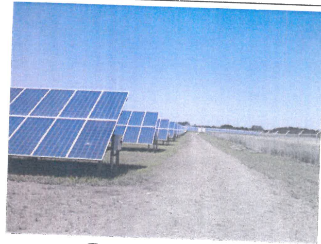
Front View of Array Access Road, Fence, Vegetation
