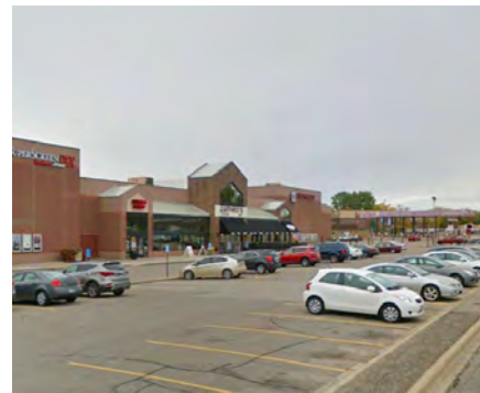
Businesses on Frontage Road N
