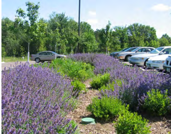
Rain gardens reduce flooding and increase green areas while remaining low maintenance. This can be a great opportunity to reduce asphalt on parking lots.
