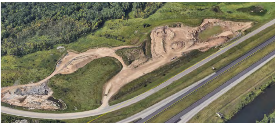
Aggregate mining site along Graniteview Road, on the eastern edge of Waite Park.
