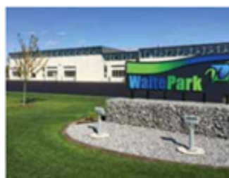
Public Works Building
