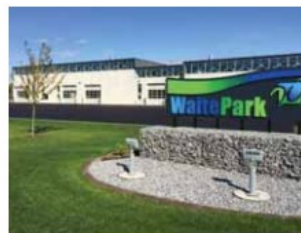
Public Works Building
